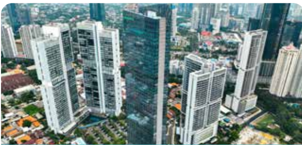
Office Tower - Ciputra World 2 Jakarta
